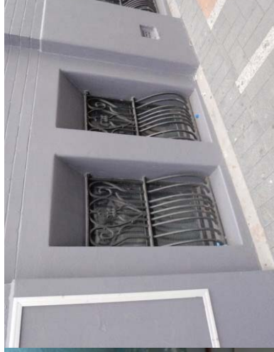
Existing metal window screens
