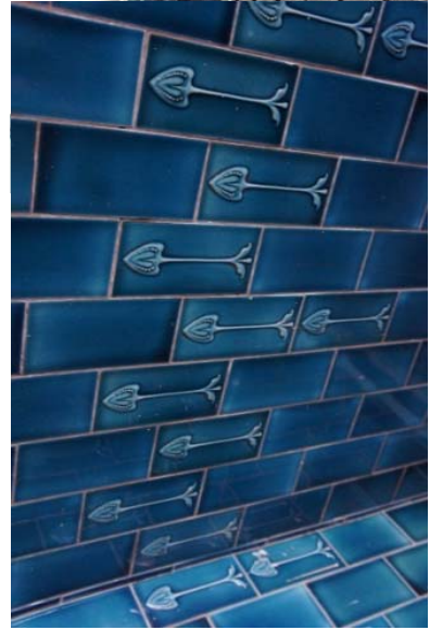
Existing tiles to original stair
