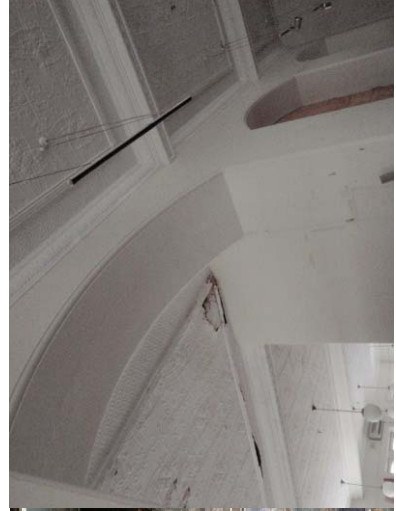
Existing structural arches + columns
